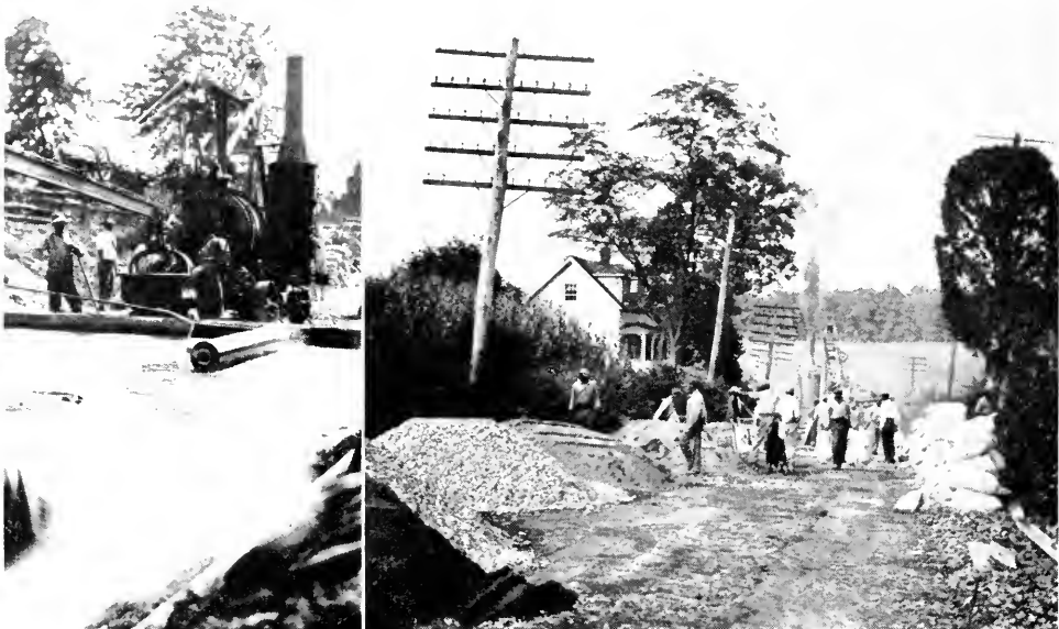
The Roads Commission met the problem by rebuilding and widening the roads with concrete shoulders. Here are typical construction scenes during and after World War I.
